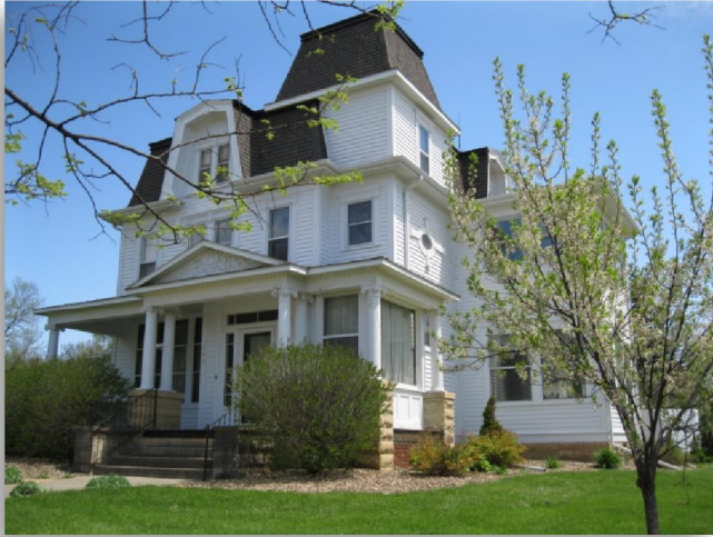
Michael Lehrer's house at 203 N. Van Buren Ave. is a good example of the Second Empire style
