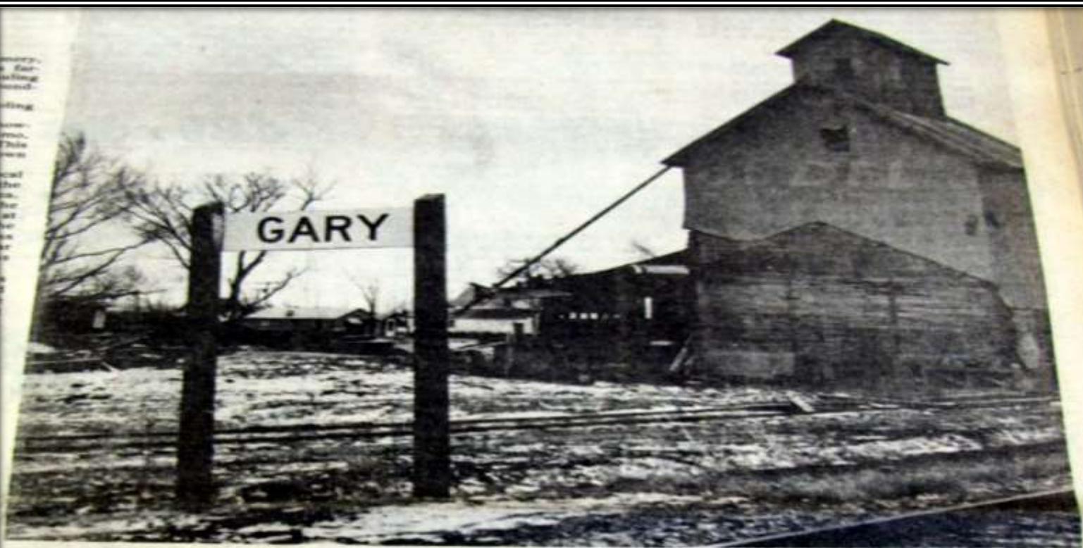
The elevator in Gary in the process of demolition.
