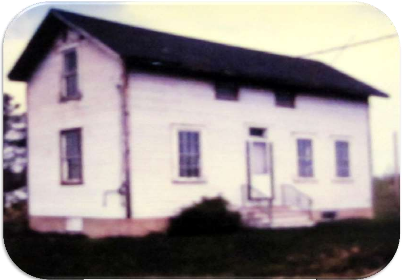
1886 Northern Pacific Section House
